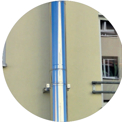
Fixings for chimneys
